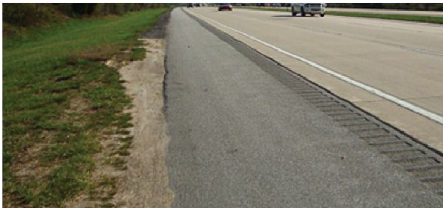
FIGURE 9 – EXAMPLE OF VISUALLY CONTIGUOUS PAVED TRAVELED WAY AND A PAVED SHOULDER Source: http://www.deldot.gov/information/community_programs_and_services/DSHSP/roadway_departure_crashes.shtml
