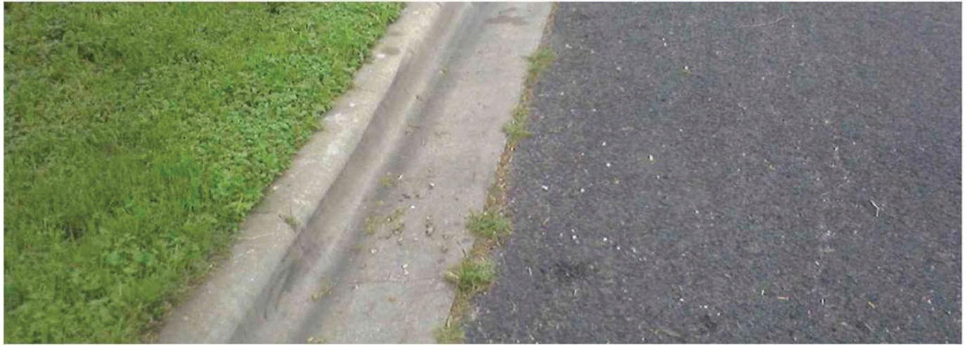
FIGURE 10 -- EXAMPLE OF A U.S. URBAN TRAVELED WAY WITH A GUTTER AND CURB Source: http://collegetri.files.wordpress.com/2012/06/curb-of-a-road.jpg
